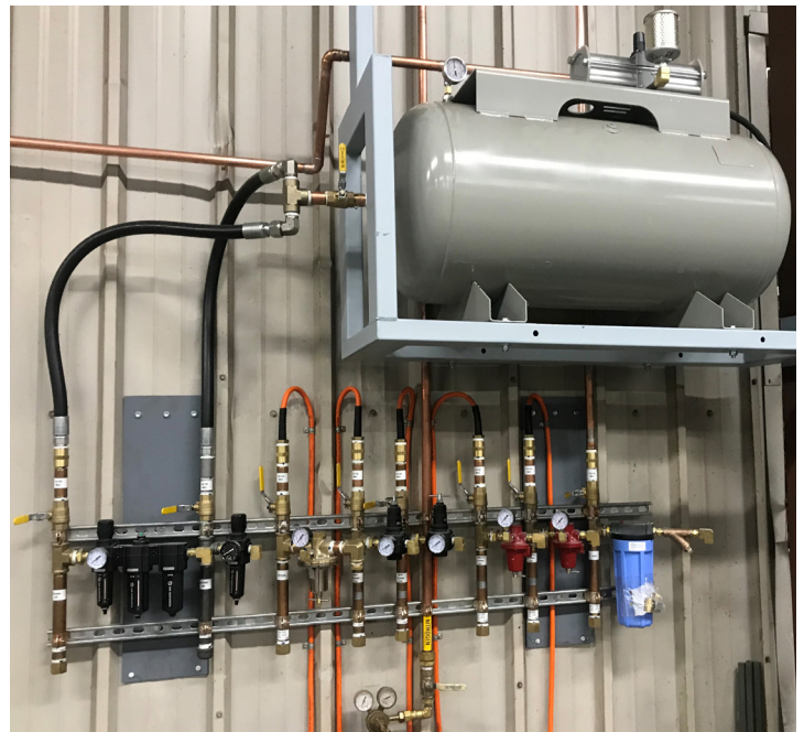
Customer mounted plasma station equipment. Also showing an optional plasma air booster tank. (Mounting hardware by customer.)
